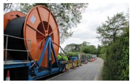
Figure 4.13: Cable Drum at Joint-bay location
